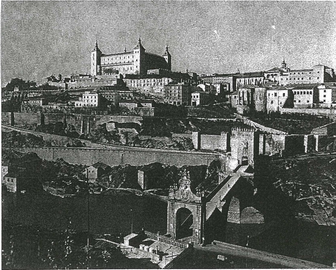
View of Toledo, Spain, with the Alcántara Bridge over the Tagus River
